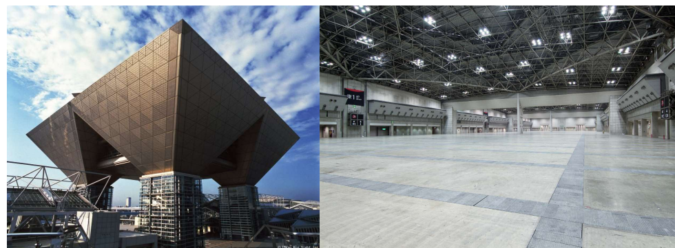
Tokyo Big Sight (6) Electrical Facilities Work for Renovation of the East Exhibition Building
