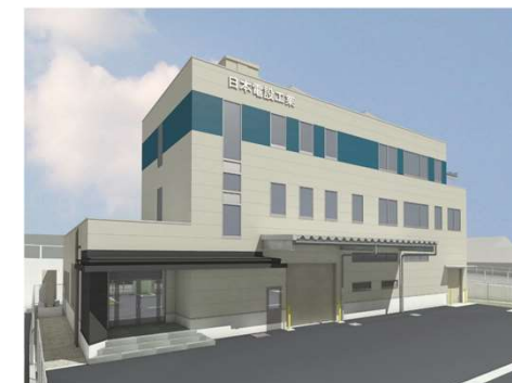
NDK Nagano Building (under construction)
