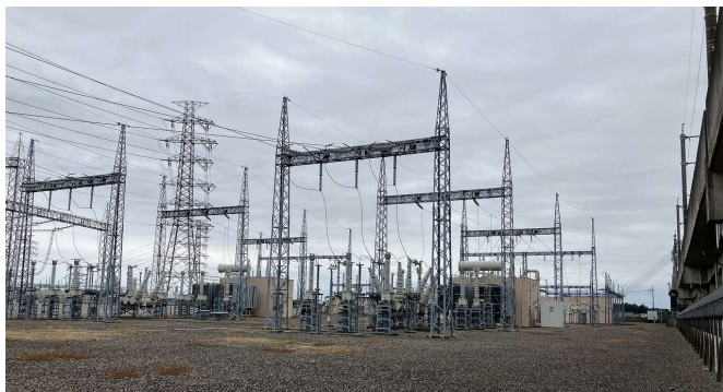
Work to Replace Panelboards and Other Work at Six Locations on Tohoku Shinkansen, including Shin Utsunomiya Substation
